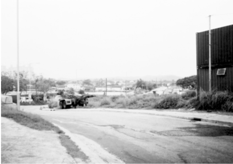
Access road branching off Fuk Shun Road
