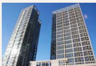
Tianjin Hailrun Plaza
