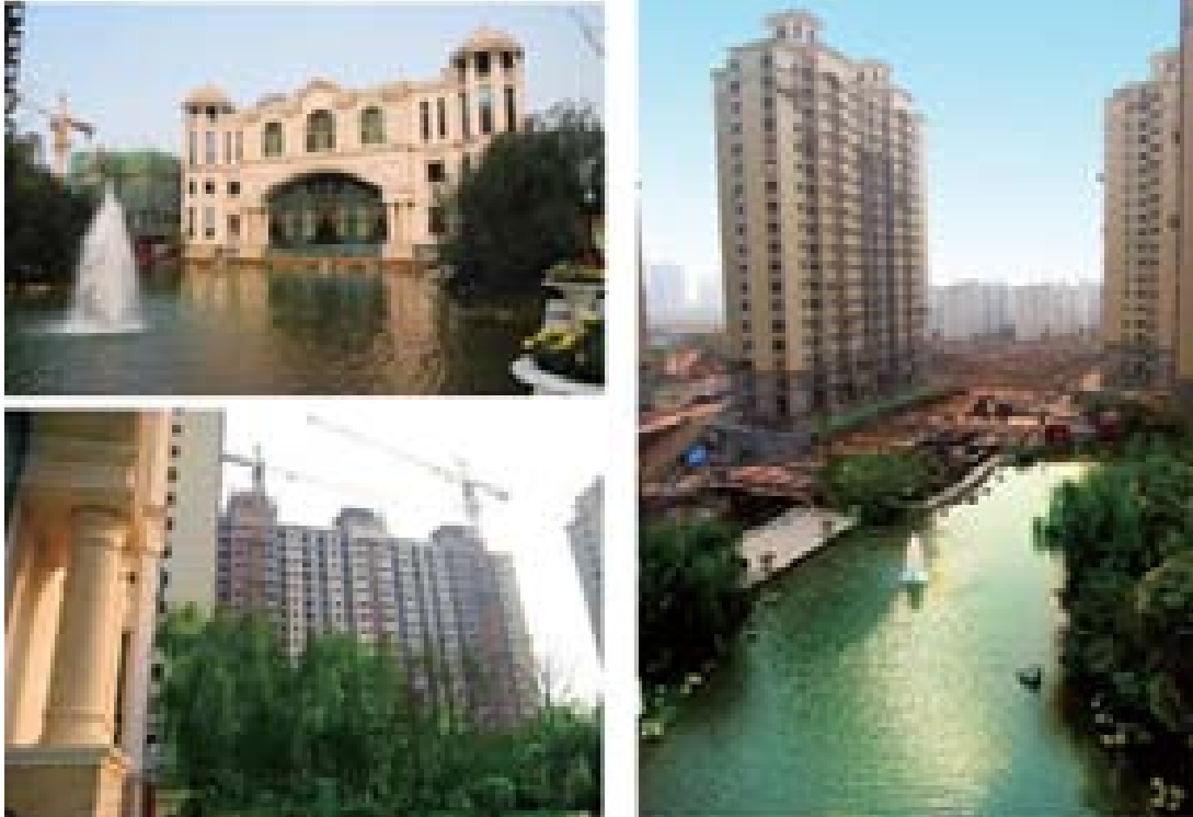
Construction Site and Garden View of Evergrande Metropolis Xi'an Phase 1
