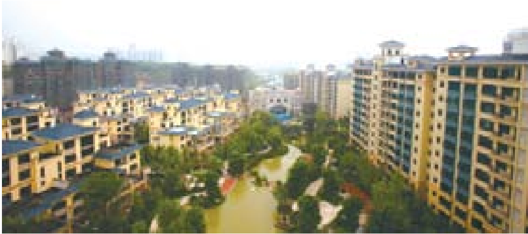
Construction Site of Evergrande Palace Chongqing Phase 1
