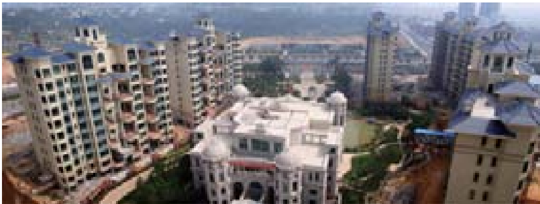
Construction Site of Evergrande Palace Changsha phase 1
