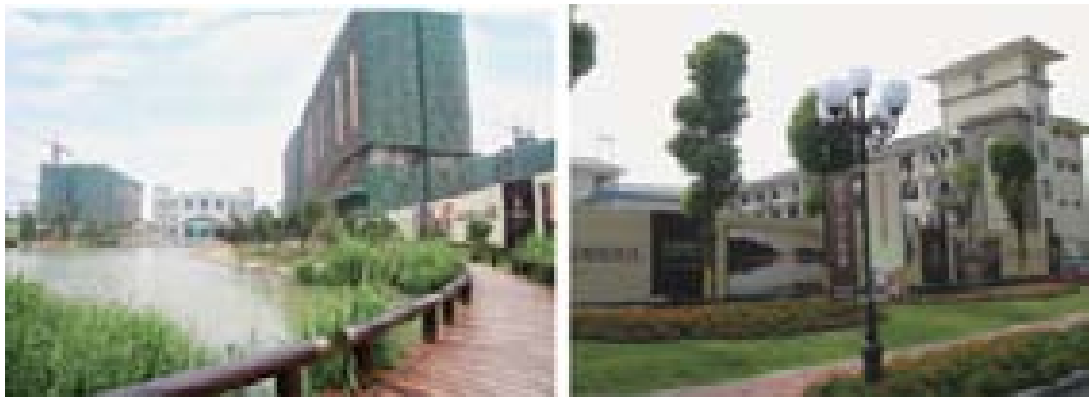
Facilities of Evergrande Oasis Wuhan
