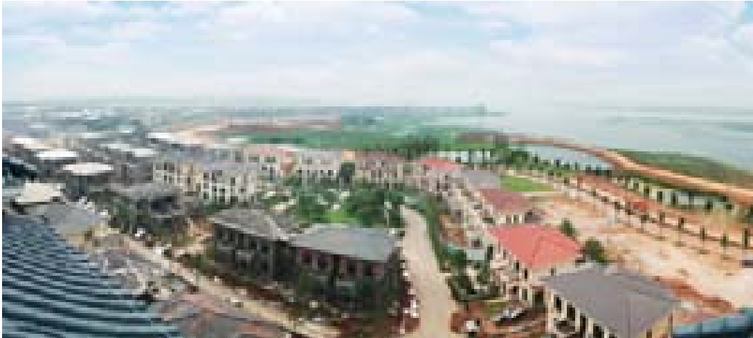
Construction Site of Evergrande Splendor E'zhou Phase 1
