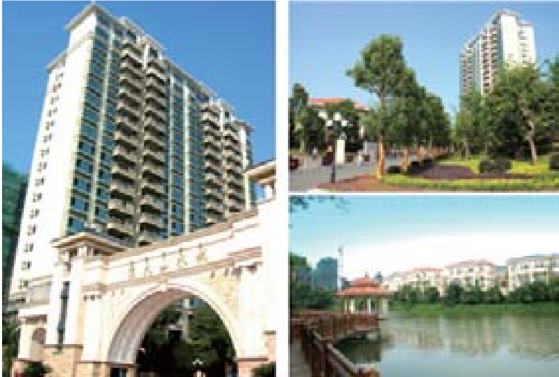
High-rise Residential Buildings and Garden View of Evergrande Scenic Garden Phase 1
