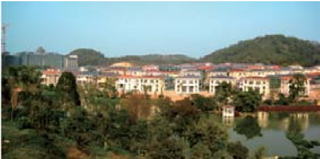
Construction Site of Villa of Evergrande Scenic Garden
