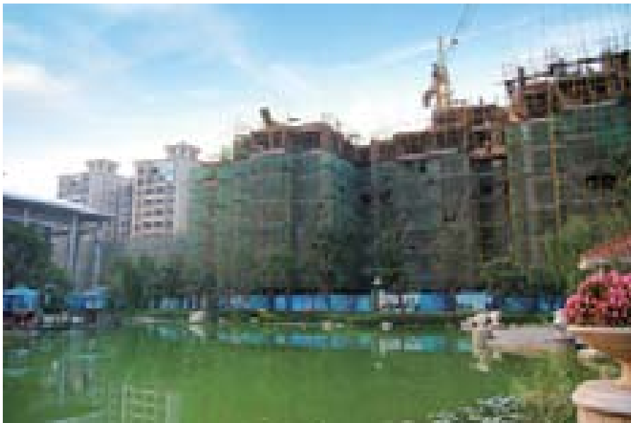
Construction Site of Evergrande Oasis Xi'an Phase 1
