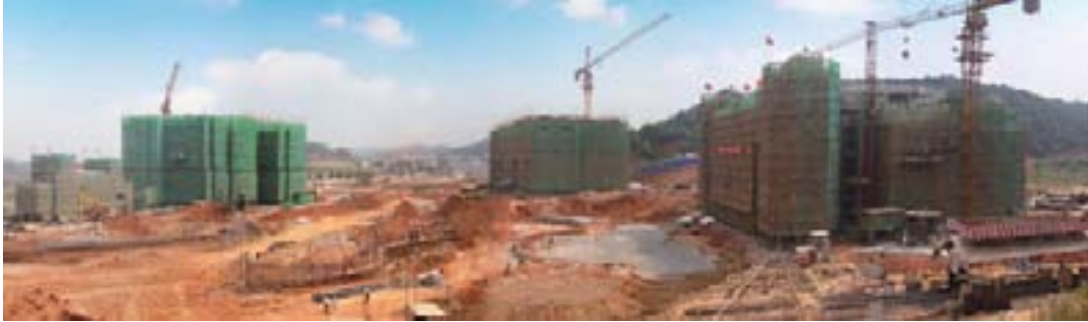
Construction Site of Evergrande City Changsha Phase 1
