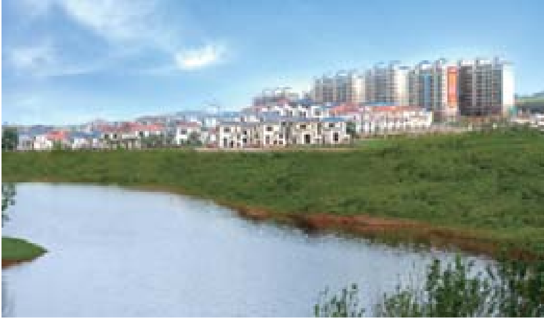
Construction Site of Evergrande Splendor Kunming Phase 1
