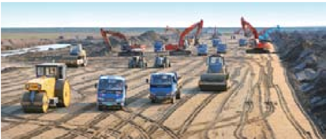
Road Construction site of Evergrande Splendor Qidong
