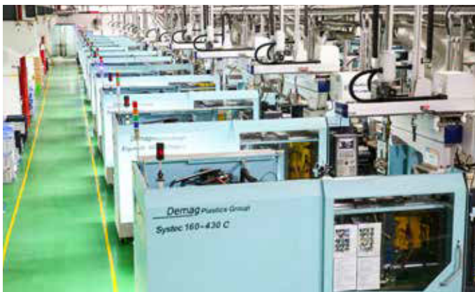
Plastic injection production lines
