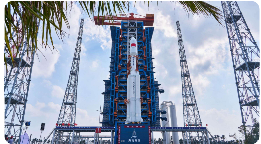
Modernized Rocket Launch Pad
