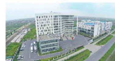
Qidong Offshore Hydrogen Energy Business Division
