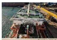
Gas Supply & Liquid Cargo System
