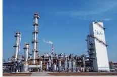
Liquefaction plant for natural gas, coal-bed methane and coke oven gas
