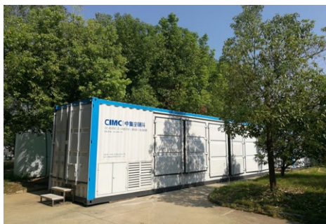
Container Type Garbage Leachate Treatment Device
