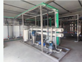
Filtration and Recovery Unit at the Wastewater Station
