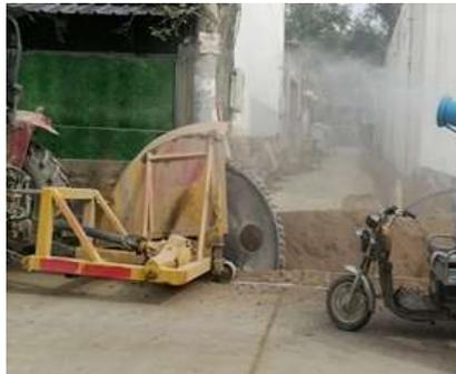
Replace excavators with grooving machines in part to reduce construction costs
