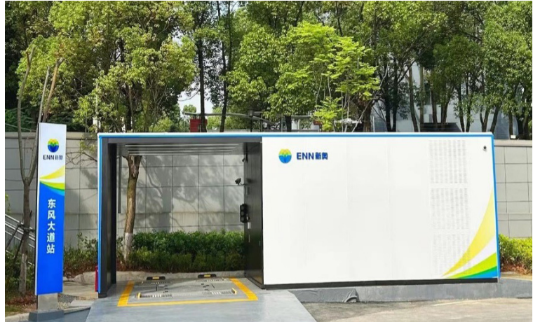
ENN Energy Operated Autonomous Driving Battery Swapping Station
