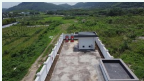
Gas Micro-Pipeline Project Facilities
