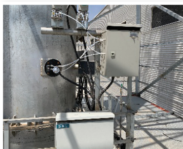
Online Monitoring System for Smoke and Gas Emission
