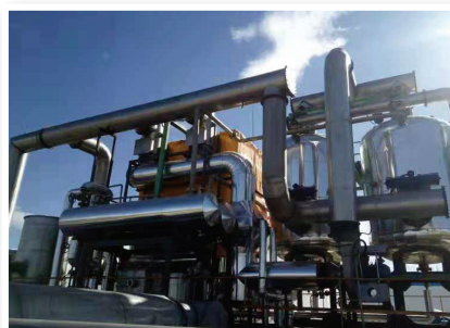
Condensed Fiber Adsorption and Regeneration System
