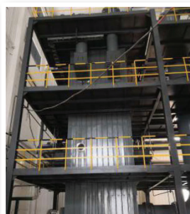
Wet Static Dedusting and Mist-eliminating Purifiers
