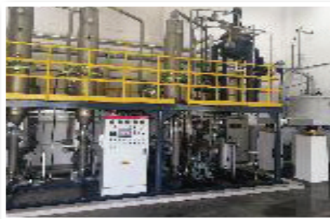
Detoxification Treatment Facility for Concentrated Ammonia Solution of Baike
