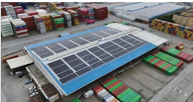
The 7.3 MW BIPV project of Guangzhou South China Oceangate Terminal
