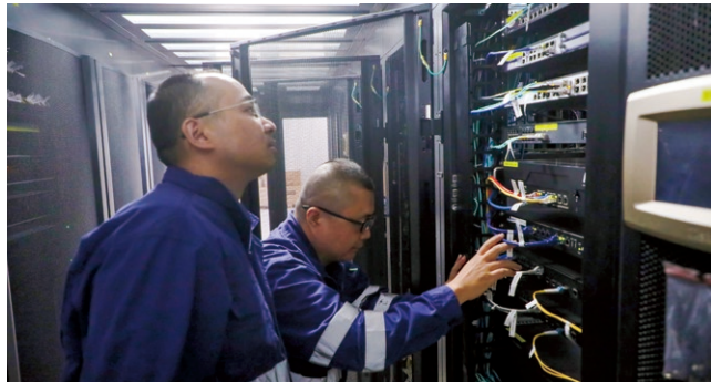
Simulated on-site troubleshooting of information malfunctions
