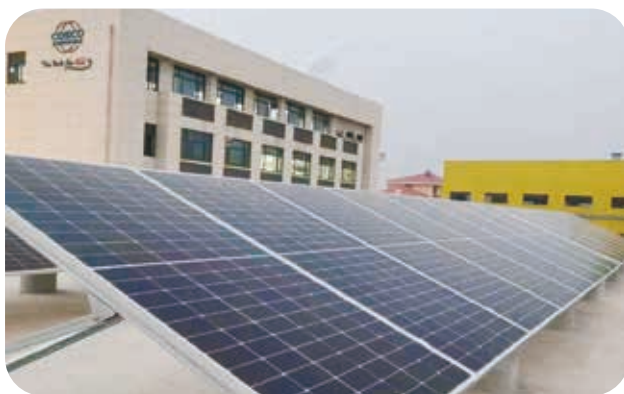
CSP Wuhan Terminal has installed 1,063 pieces of 545WP monocrystalline silicon solar photovoltaic modules on the roof of 5,768 square meters in the port area, with a designed capacity of 0.578MWp, providing clean power for the production in the port.
