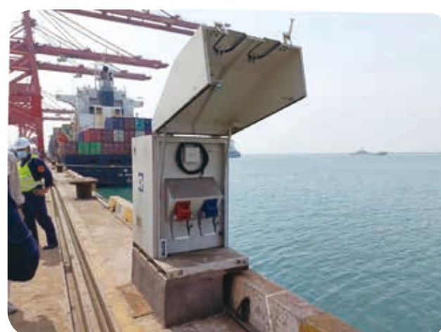
Lianyungang New Oriental Terminal completed the construction of two sets of 5MVA high-voltage shore power supply systems and supporting shore power socket boxes, and upgraded five sets of low-voltage shore power boxes to meet the needs of shore power connections for various vessels.
