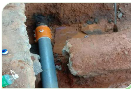
After water supply pipe maintenance
