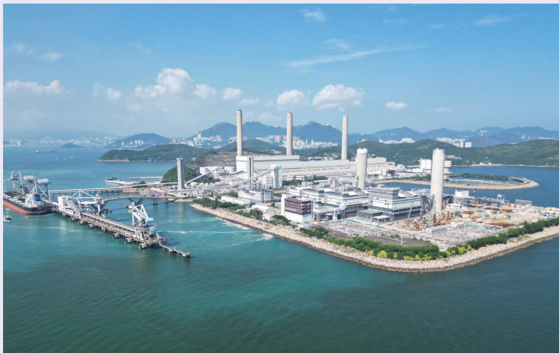
Lamma Power Station, HK Electric
