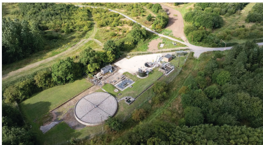
Northumbrian Water continues to upgrade its sewage networks and treatment systems.
