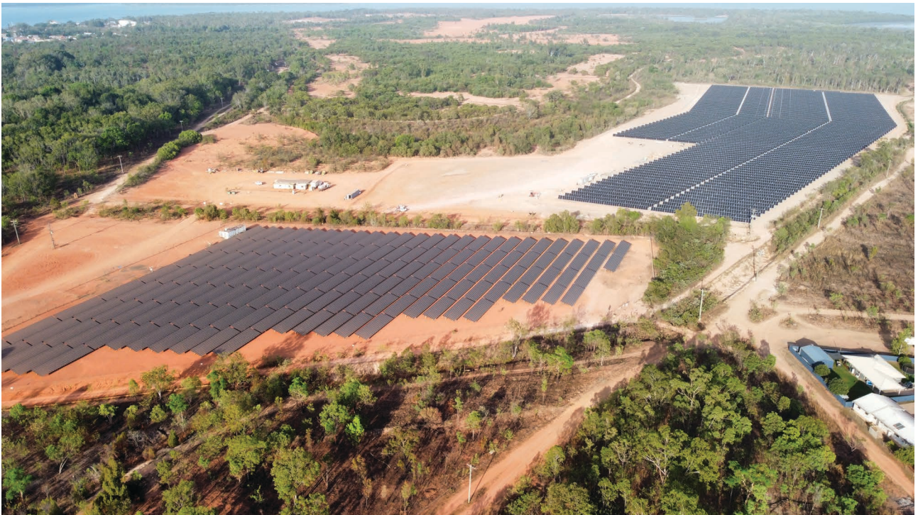
Solar panels at EDL.
