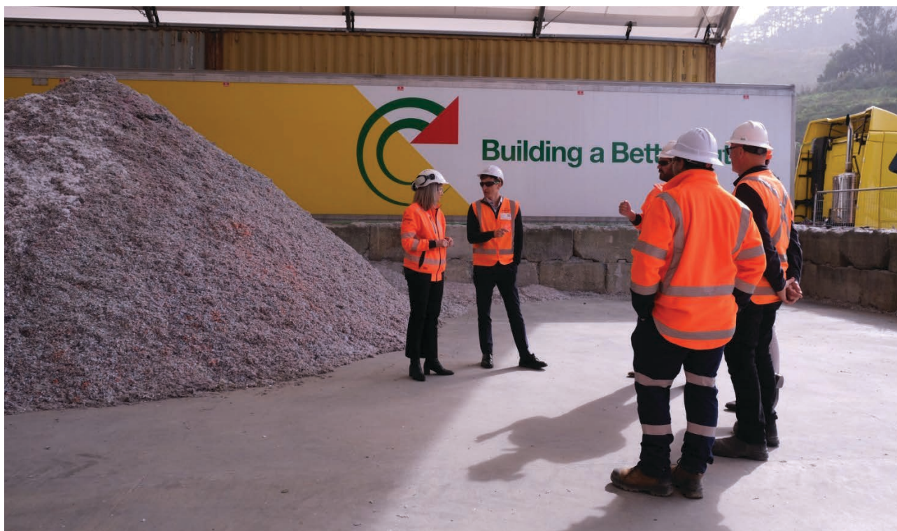
EnviroNZ commissioned New Zealand's first plant to convert unrecyclable plastics into process engineered fuel.
