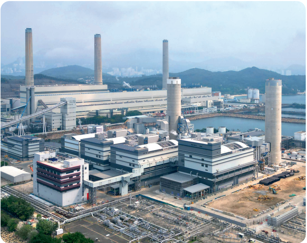
Lamma Power Station, HK Electric
