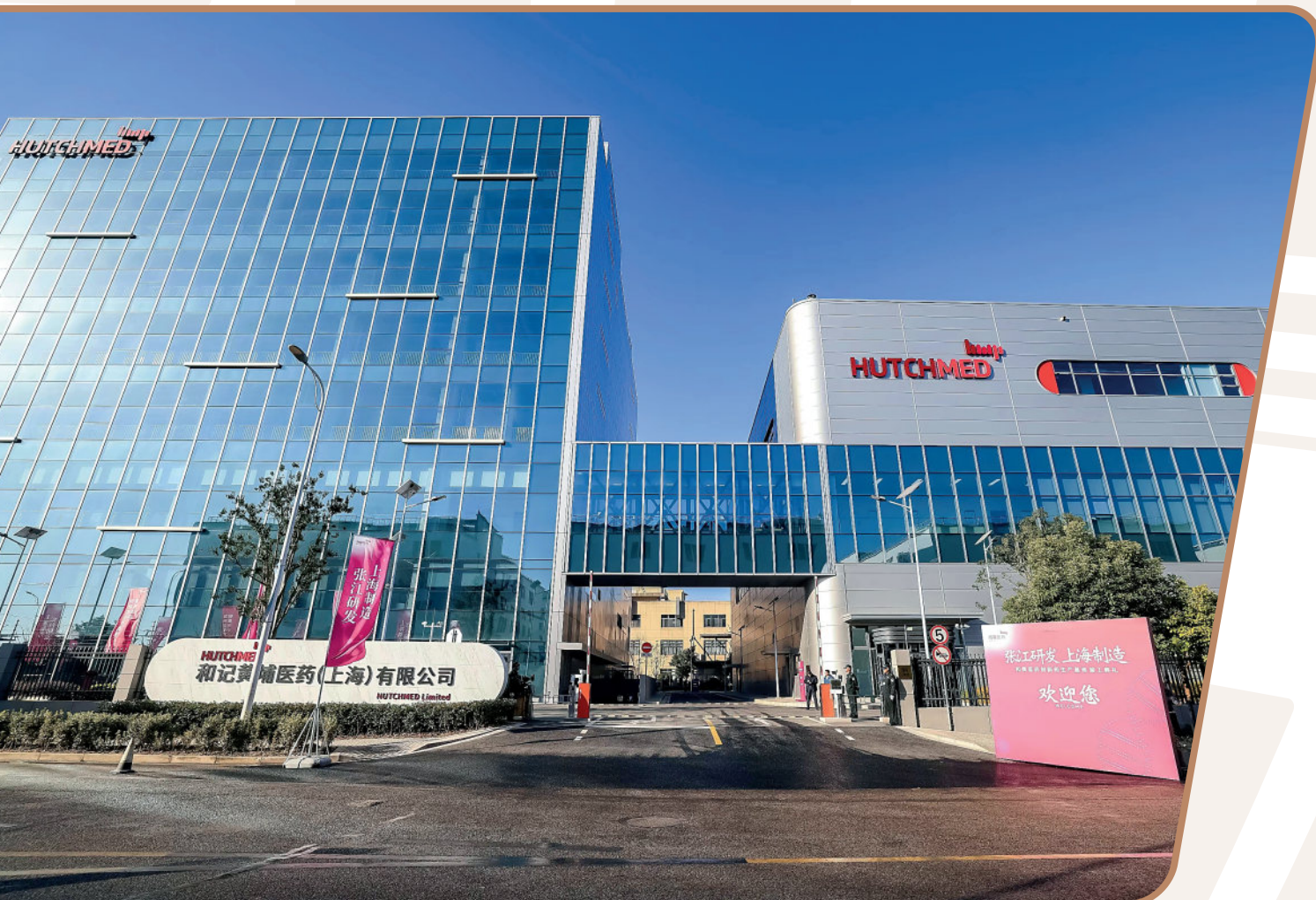
HUTCHMED's new flagship manufacturing facility in Shanghai, China, commences operations.
