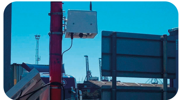
Air quality monitoring unit, Hutchison Ports UK
