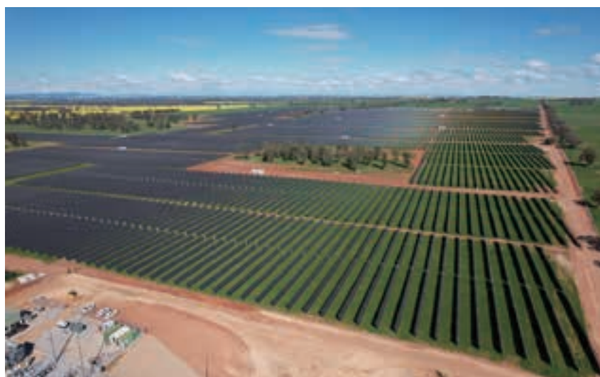
Victoria Power Networks 太陽能裝置
