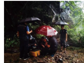
Jilin Unicom employees carry out emergency repairs in wind and rain
