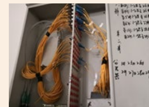
Rectification of network boxes and cable hubs.
