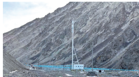
● 5G base station building a “digital sky road”
