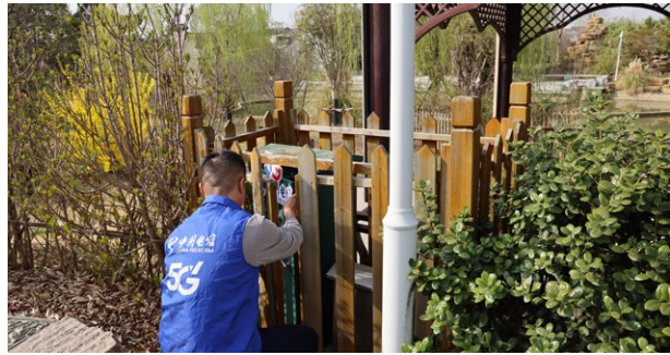
Staff conduct inspection and maintenance on communication facilities
