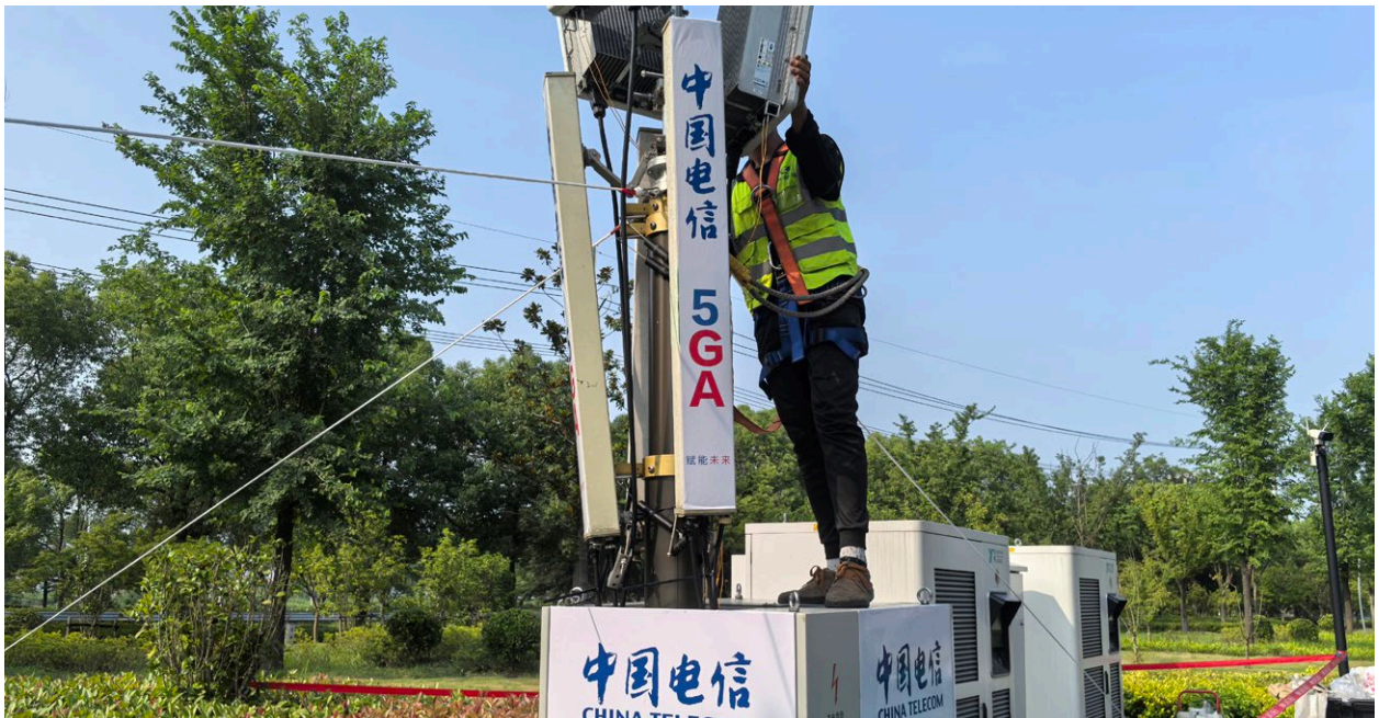
Workers are commissioning 5G base stations
