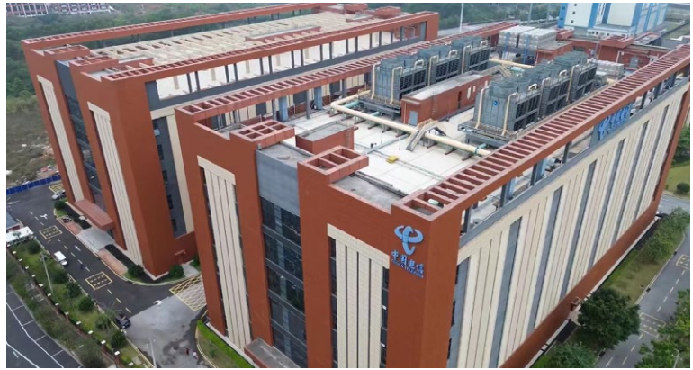
China Telecom's ASEAN International Information Park No. 2 Data Centre
