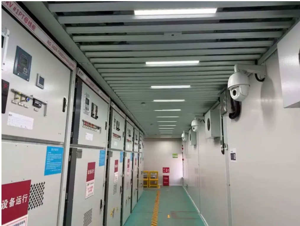
▲ Data acquisition camera in 35 kV HV switchgear room
