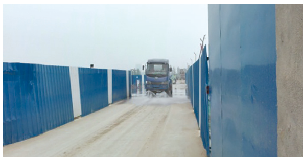
The construction site was enclosed and water spray was used to suppress dust
