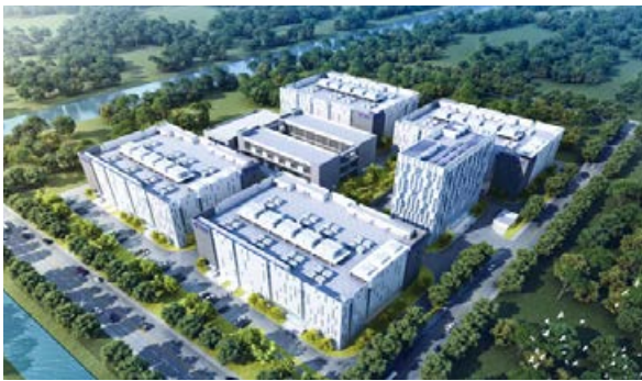
● Wujiang Computing Power Center, Eight National Computing Hubs
