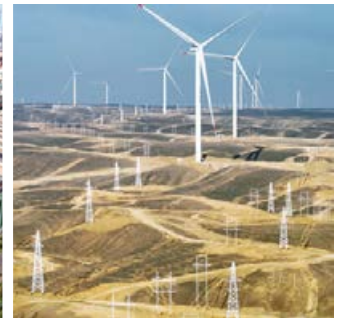
Hami Wind Storage Supervision Project
