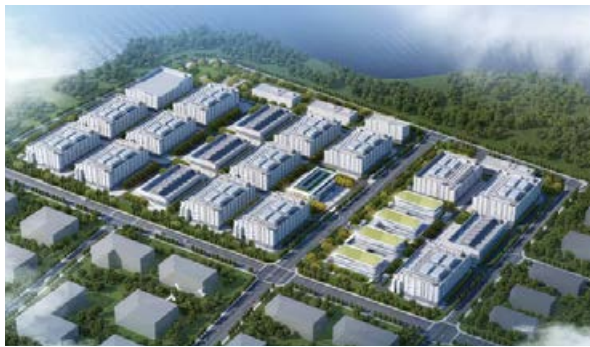
● General Contracting Construction Project of a Central Big Data Center (Cybersecurity Base)
