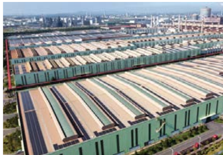
Rooftop Distributed Photovoltaic Project for a Steel Company in Qingdao
