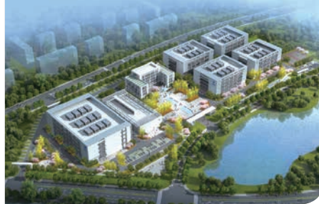
China Telecom (National) Digital Qinghai Green Big Data Center Project
