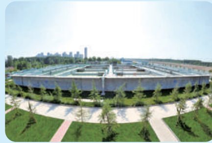
Ji'nan Waste Water Treatment Project 濟南污水處理項目 (Overall site greenery area: approximately 94,000 m 2 ) (整體廠區綠化面積：約94,000平方米)
