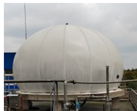
The double-film biogas bag was replaced
