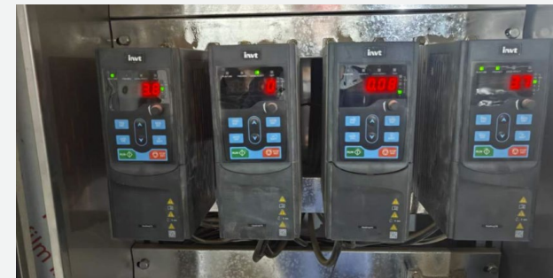
Renovation of Water Supply System
