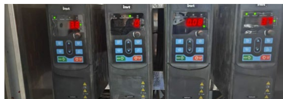
Water Supply System Renovation
