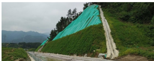
Revegetation of Access Road Slopes at Shiyan Project Site
