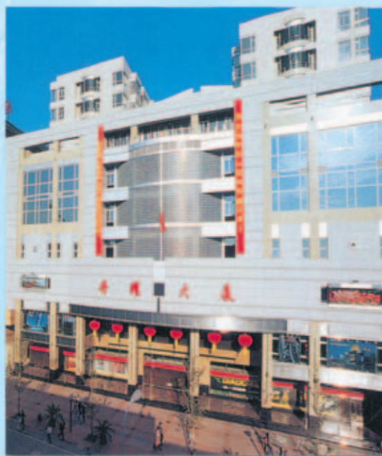
Danyao building erected on Lot No. B3 of the Wangfujing Project
