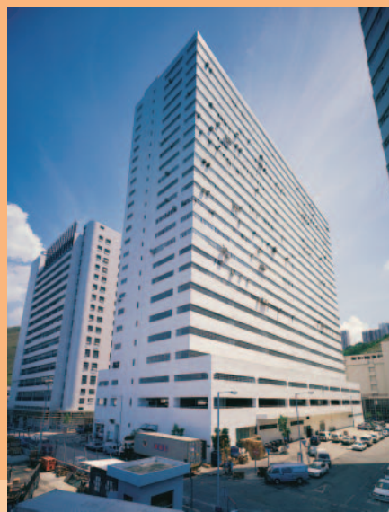
Harbour Industrial Centre, Ap Lei Chau, Hong Kong
