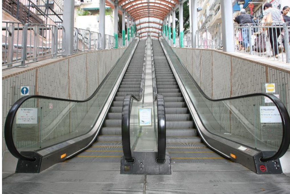
Provision of Universal Accessibility Facilities at Footbridges, Elevated Walkways and Subways
