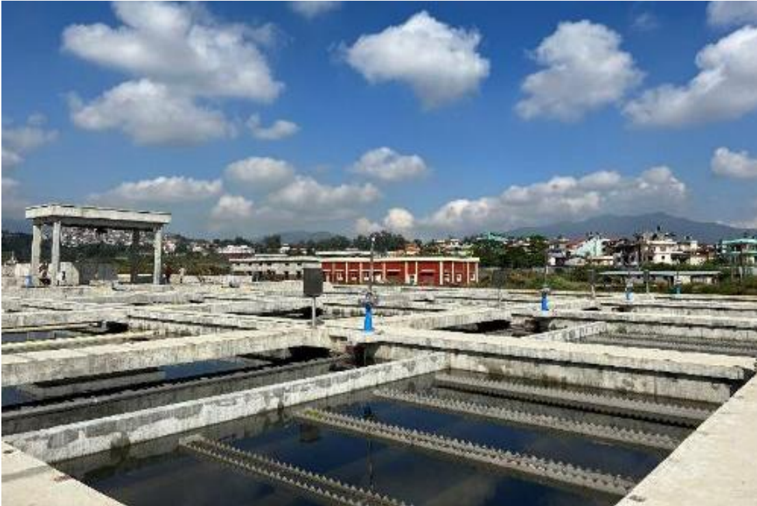
Dhobighat Wastewater Treatment Plant, Nepal
