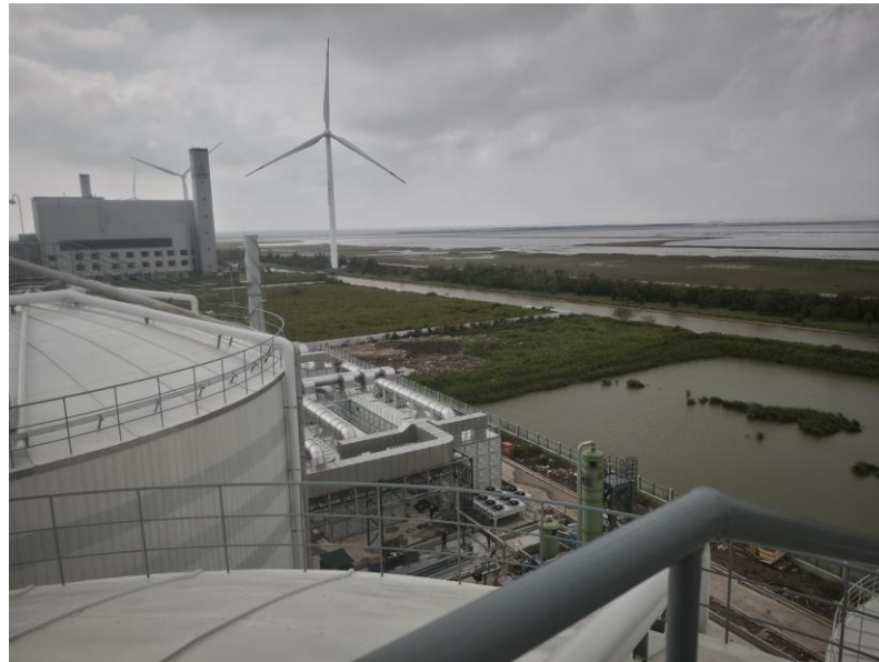
Combined Heat and Power, Shanghai Chongming
