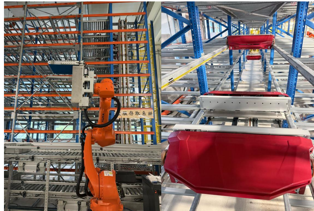
Supply and installation of Automatic Storage & Transportation System for Hospital Authority Services Centre
