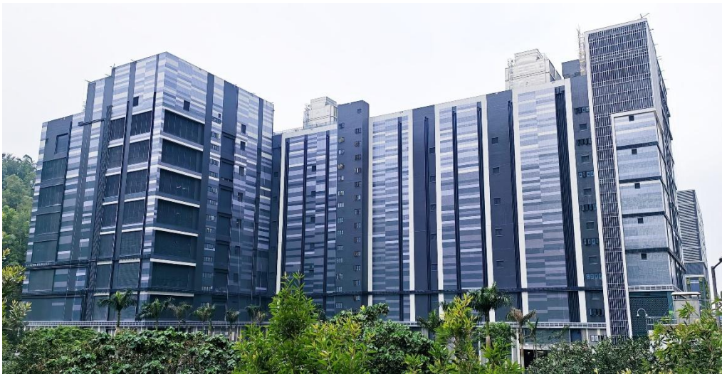
Data Centre Fitting-out Work for a Major Data Centre Service Provider in Tseung Kwan O
