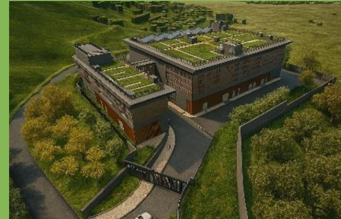
San Shek Wan Sewage Treatment Works
