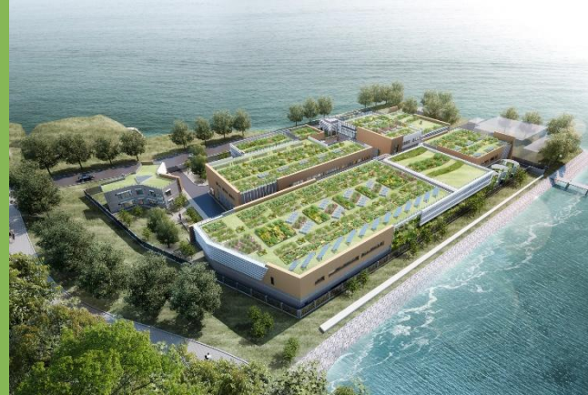
Cheung Chau Sewage Treatment and Disposal Facilities
