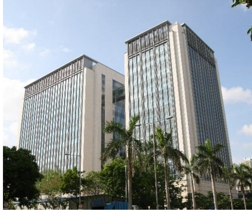
West Kowloon Law Courts Building
