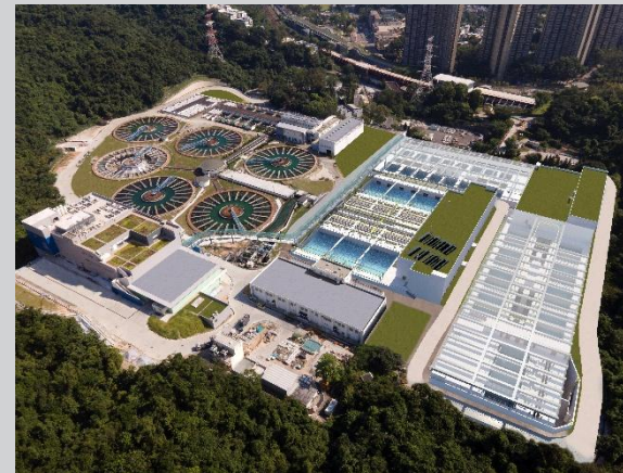
In-situ Reprovisioning of Sha Tin Water Treatment Works
