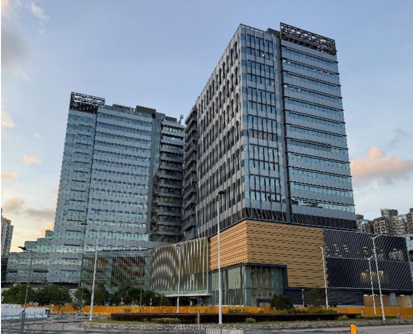
Joint-user Government Office Building in Tseung Kwan O
