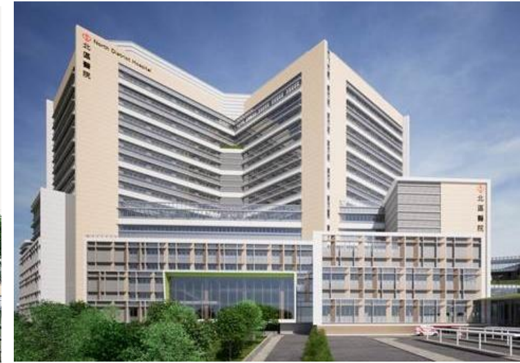
Expansion of North District Hospital
