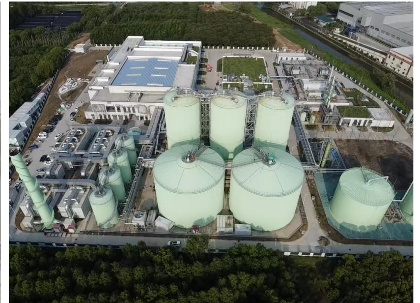
Combined Heat and Power, Shanghai Qingpu
