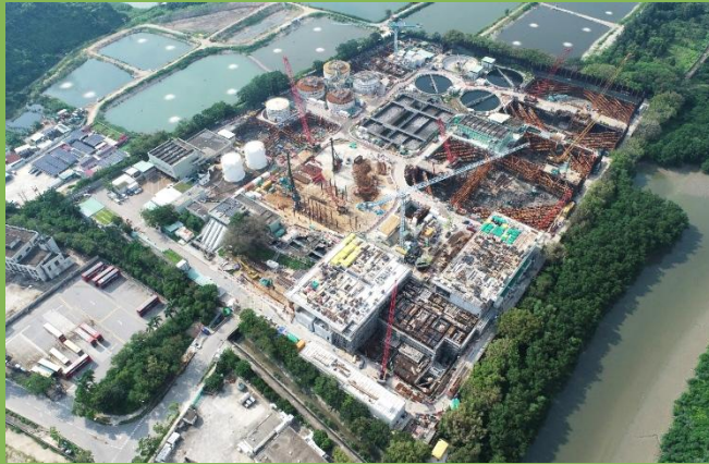
Yuen Long Effluent Polishing Plant
