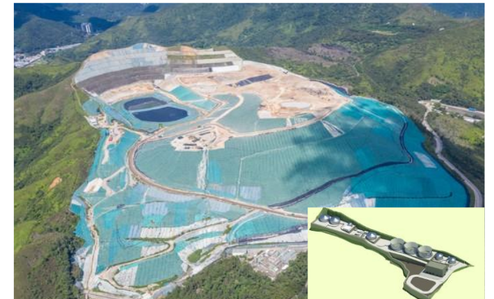
New Leachate Treatment Plant for North East New Territories Landfill Extension (NENTX)
