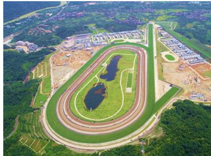
Hong Kong Jockey Club Conghua Racecourse Training Centre Phase I and Phase II, Mainland China
