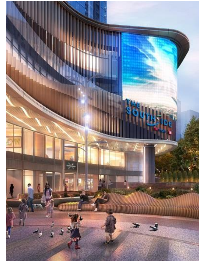
Supply and Installation of CCTV Systems with Video Analytics for Southside Mall, Wong Chuk Hang
