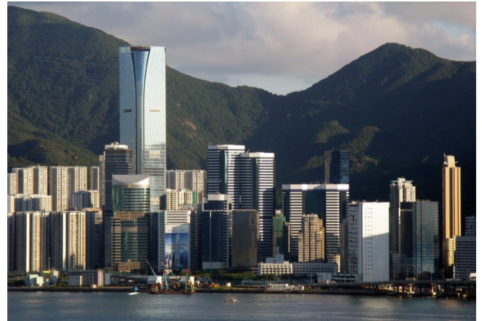
Supply and Installation of Access Control Systems in Taikoo Place
