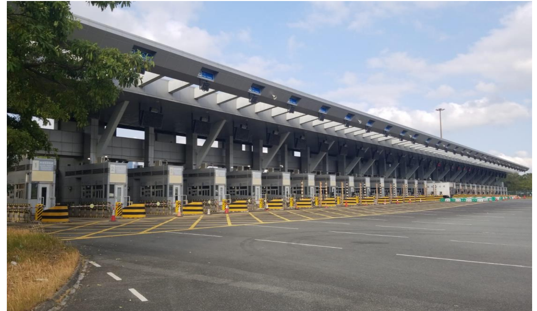
Supply and Installation of Automatic Vehicle Clearance Support System in Shenzhen Bay Control Point
