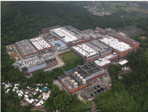
One of our projects involves expanding the existing water treatment and pumping facilities at a water treatment plant in Tai Po to increase its output capacity from 400,000 m<sup>3</sup>/day to 800,000 m<sup>3</sup>/day. This will enhance the reliability and flexibility of the water supply and distribution system in the freshwater supply zone of Tai Po.
