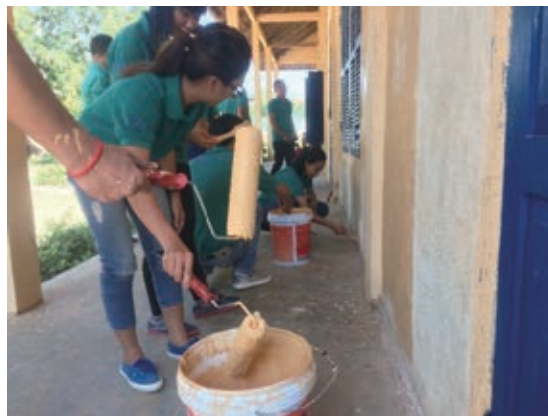
Painting walls at Prey Tbes Primary School
