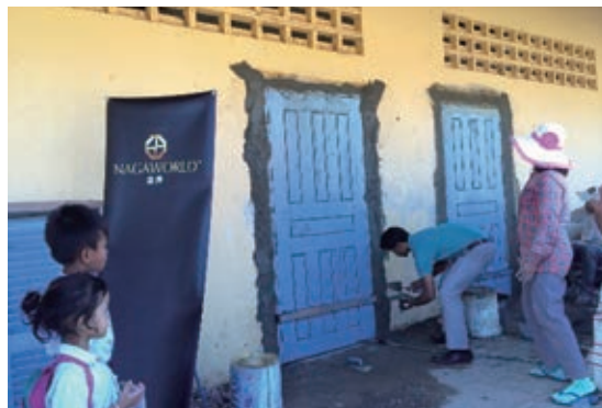
Replacing doors and windows at Hun Sen Chibal Primary School
