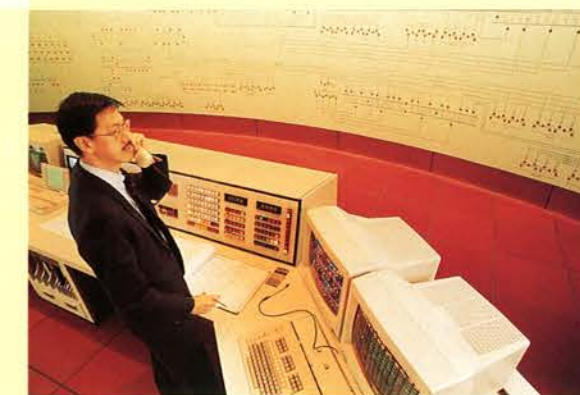
The System Control Centre at Hongkong Electric's headquarters monitors all facets of the company's supply network.
