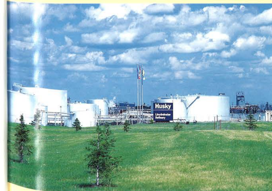
Husky's Refinery at Lloydminster processes heavy crude oil into asphalt products. The refinery has a throughput capacity of 25,000 barrels per day.
