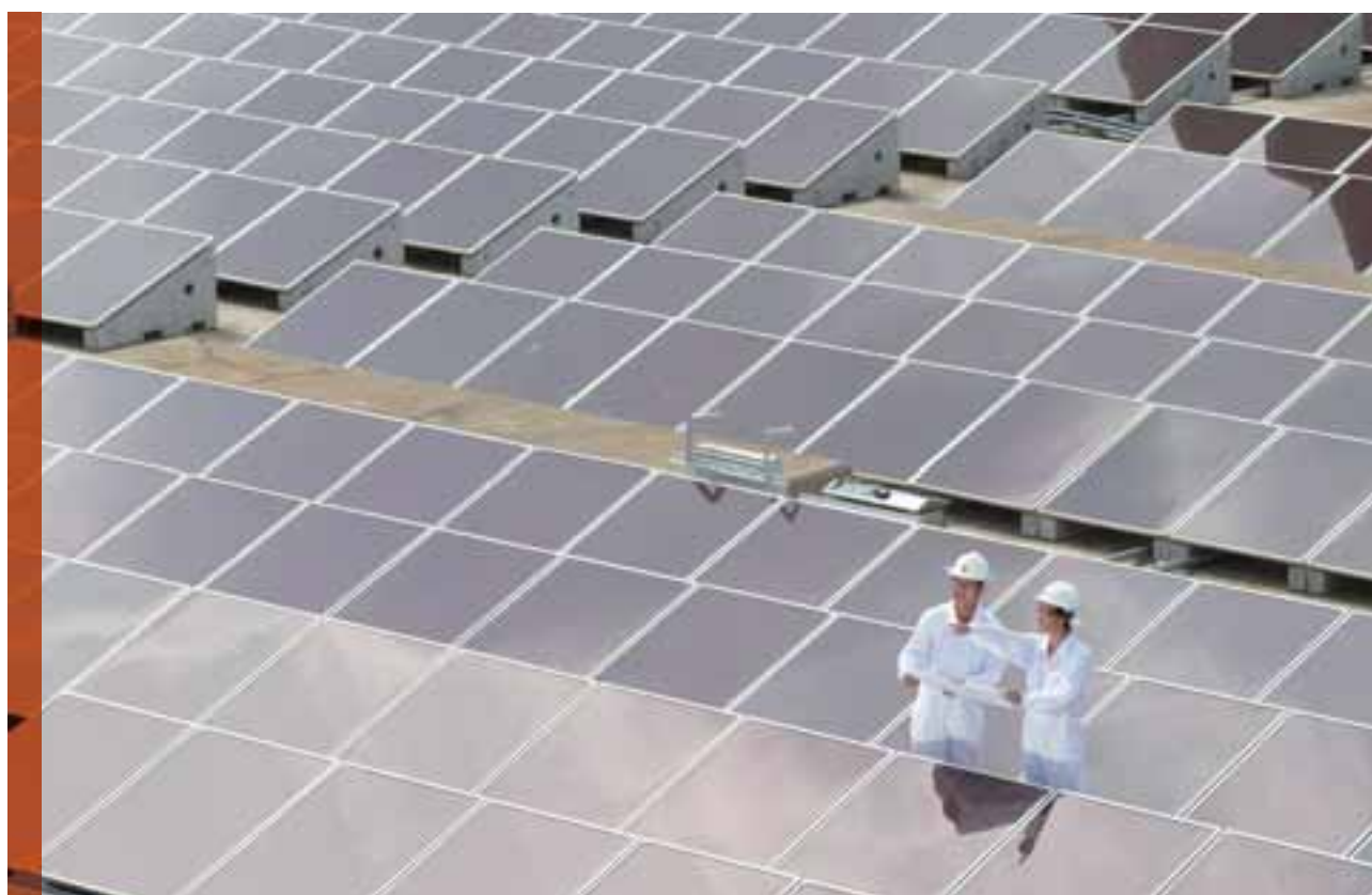
HK Electric commissions Hong Kong's largest solar power system at Lamma Power Station, which comprises 5,500 photovoltaic panels.
