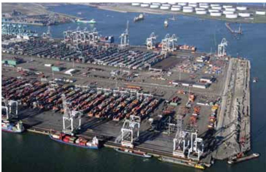
● Construction of the new Delta Barge Feeder Terminal is underway at the tip of the ECT Delta Terminal.
