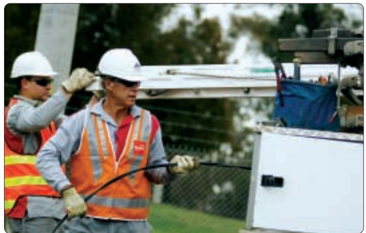
● Powercor lineworkers complete a task as part of Powercor's comprehensive network maintenance programme. The Powercor network is the largest in Victoria, covering 65% of central and western Victoria with more than 640,000 customers.
