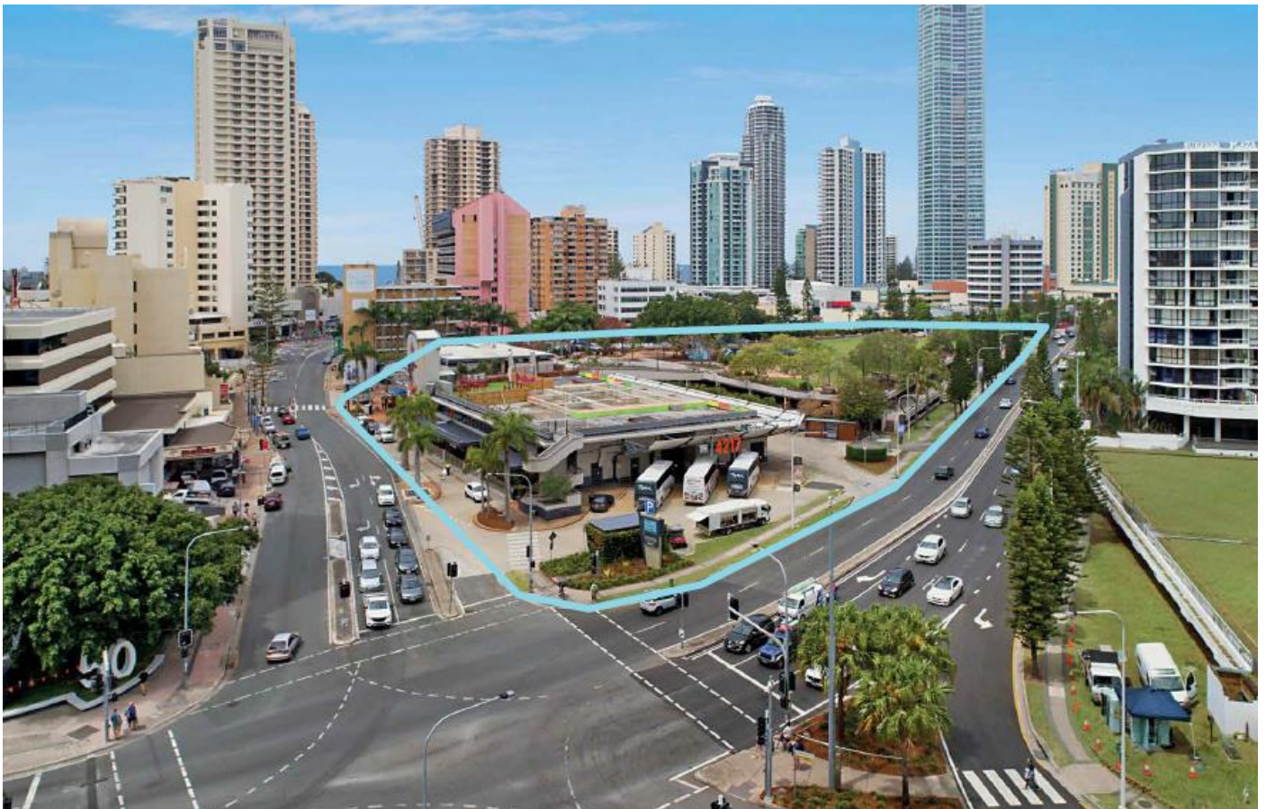
Photo caption: the Surfers Paradise Transit Centre and Bruce Bishop Car Park in Gold Coast is a fully automated car park consisting of 1,545 bays, with freehold site area of approximately 1.8 hectares.
