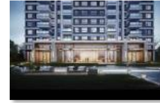
Chengdu Yinweilai Land acquisition: Dec 2019 Project launch: Aug 2020
