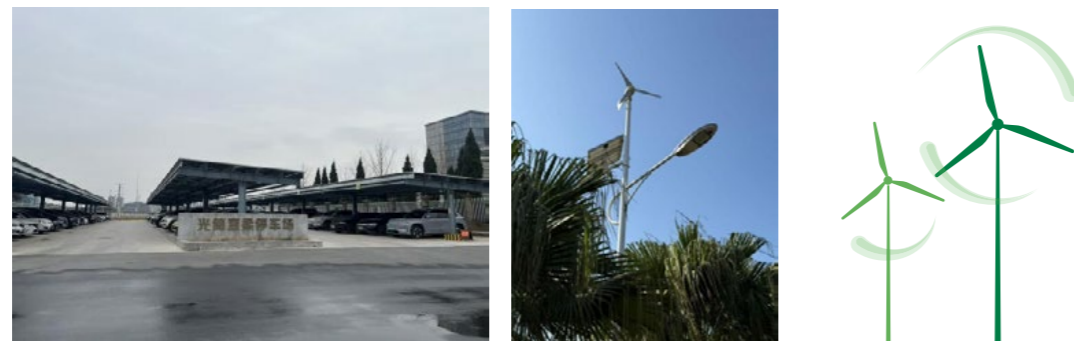
Photovoltaic-Storage-DC-Flexible Parking Lot (Left) and Wind-Solar Complementary Streetlights (Right)
