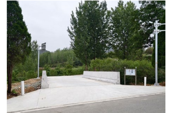
Shandong Company Assisted in Infrastructure Construction in Wulian County, Rizhao City
