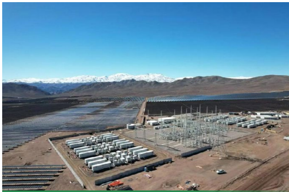
XYZ Storage Chile 117MW/262MWh Energy Storage Project
