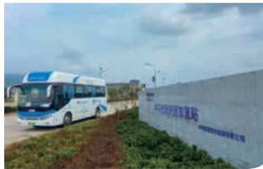
Zhongguancun Yanqing Hydrogen Refueling Station
