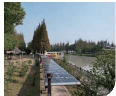
Integrated Intelligent Energy Project of CP Changxing in Jiangxiang Village
