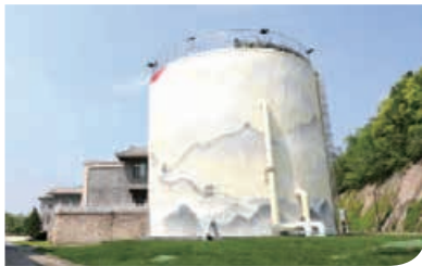
Baozhigu Integrated Intelligent Energy Demonstration Project
