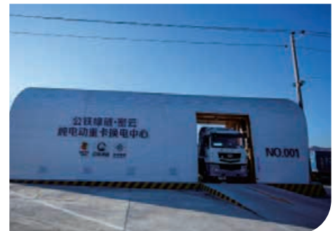
Battery swapping station for electric heavy trucks
