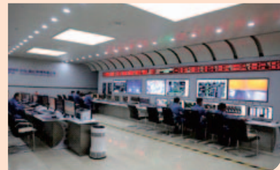
Centralised control room and power generating units at Shangqiu Power Plant maintained safe and stable operation
