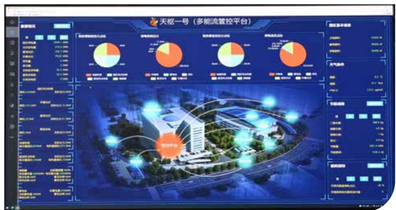
The Integrated Intelligent Energy Demonstration Project in the Office Park of Wu Ling Power's headquarters
