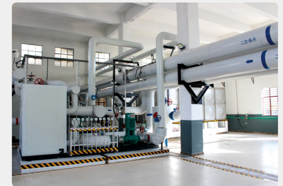
• Commissioning of water supply booster station for staff living area of Yaomeng Power Plant
