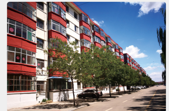
• Clean and tidy staff living area of Shentou Power Plant after renovation
