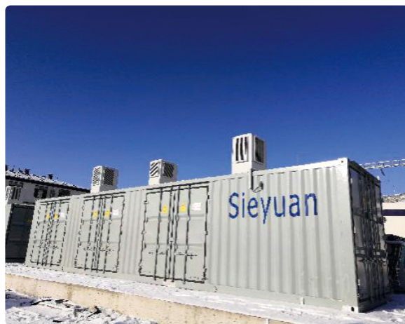
• Chaoyang photovoltaic power project: Use of container type SVG for land saving
