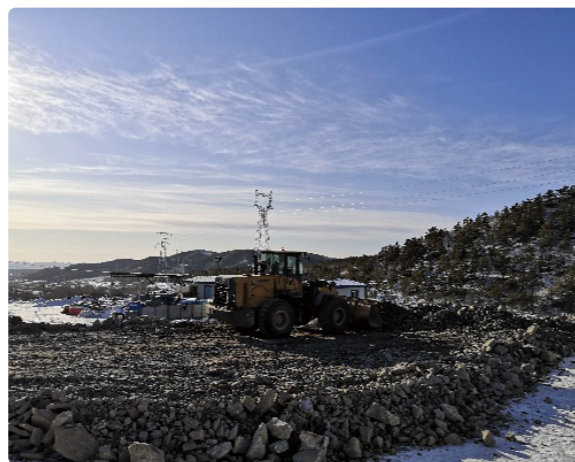
• Chaoyang photovoltaic power project: Use of waste materials and slag in road pavement for material saving
