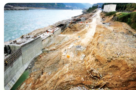
The 500MW expansion project of Wu Qiang Xi Power Plant
