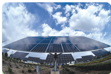
"Top Runner" photovoltaic power projects of Datong Phase II
