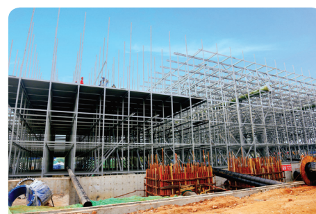
The project of upgrading Yaomeng Power Plant's water circulation
